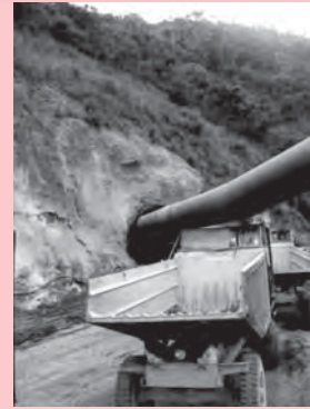
Building an Ethiopian hydroelectric power plant
